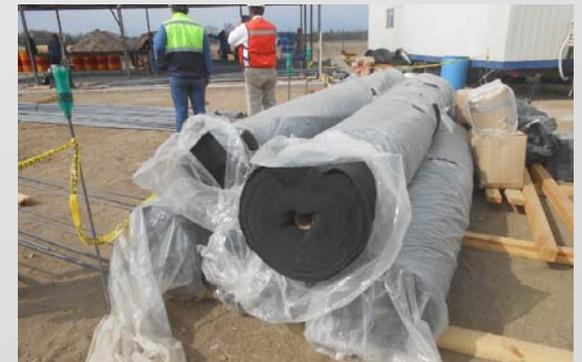
Figura 12: Geotextil
